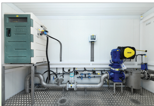
Picture 2. Equipment in wastewater acceptance unit Sewalux
