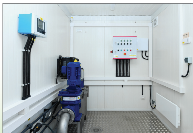
Picture 2. Equipment in wastewater acceptance unit Sewalux
